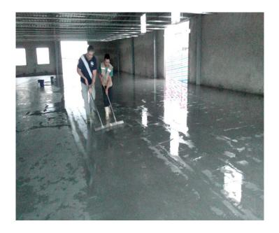
Step 2: As PENESEAL FHTM becomes slippery underfoot, lightly mist the surface with water. This will keep the material in solution providing maximum penetration. Do not allow PENESEAL FHTM to dry on the surface.
