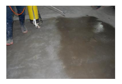
**Step 3**. Using the damp microfiber cloth and firm downward pressure, immediately spread the PENEGUARD<sup>TM</sup> (evenly, without increasing the thickness) to produce an even wet coating. Spread the product as far as possible while maintaining a wet edge. When properly applied, PENEGUARD<sup>TM</sup> dries quickly. Stop spreading once drying begins. Avoid overlapping.
