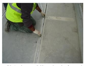
The following matrix contains the Indicative Information, regarding the desirable Width to Depth ratio (W:D) of the expansion joint, when a PENETRON® BACKING ROD is placed in the joint (The Depth is considered the distance between the surface of the joint to the surface of the backing rod).
