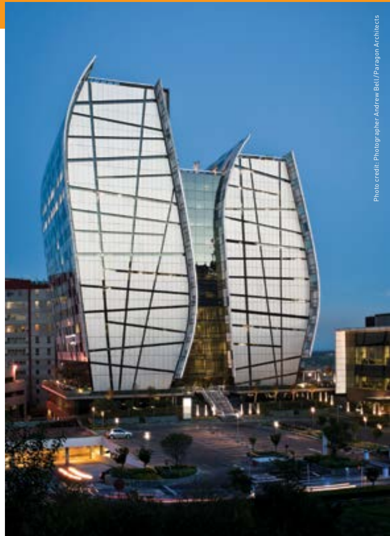
Stylish, “green” & waterproof: Alice Lane Office Towers, Johannesburg, South Africa
