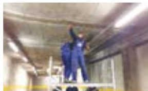
Application of PENETRON® INJECT, integral crystalline crack-injection system
