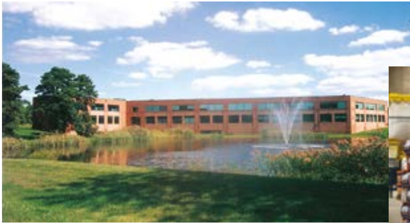
PENETRON INTERNATIONAL central offices and logistics in U.S.A.
