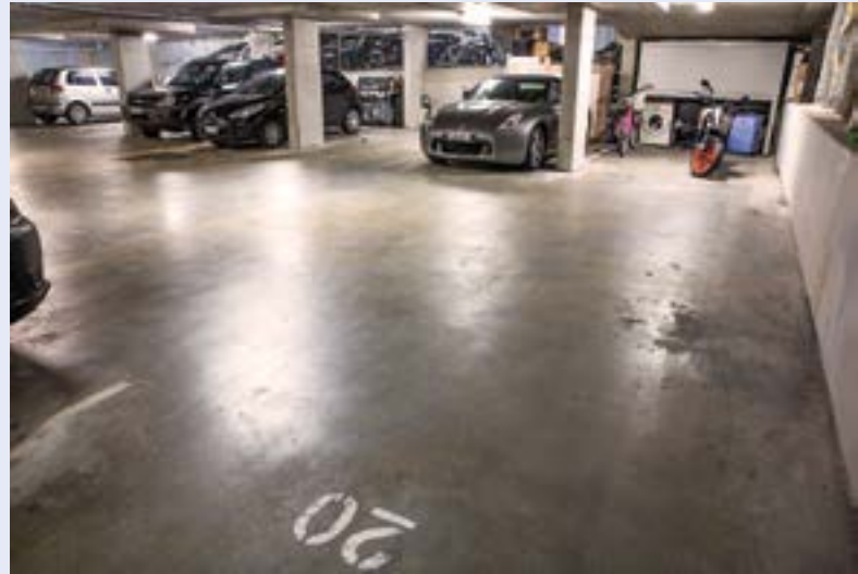
Pittwater Road Residential Parking Garage Manly, Australia
